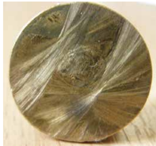
4. Complete wear of the heel ring support with rolling of the hydrostatic bearing hole
